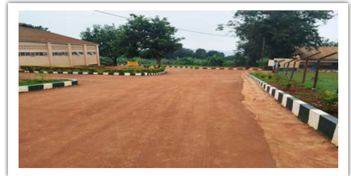
5. Completion of the lower school Tarmac
